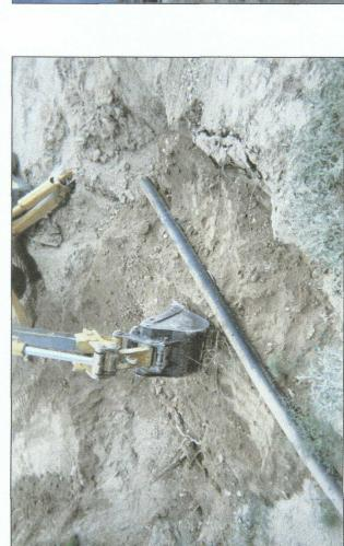
backfilling excavation and padding pipeline
