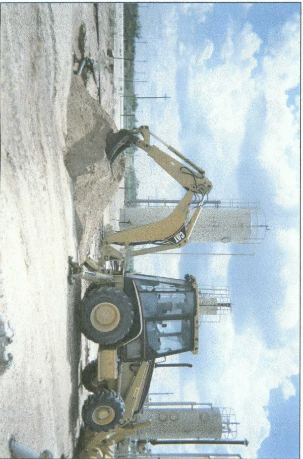
backfilling and spreading imported soil
