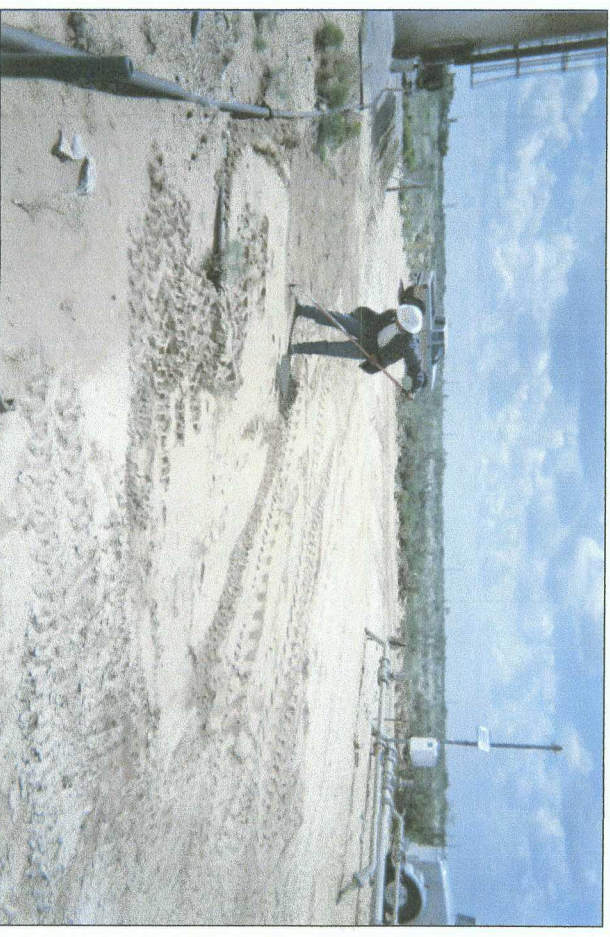
seeding backfilled area
