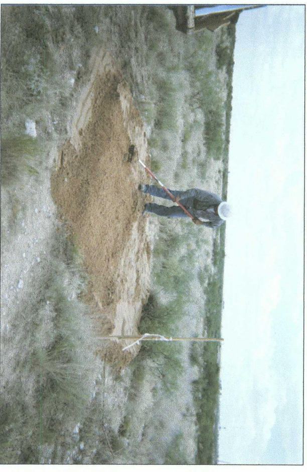
seeding at site backfilled with clean, imported soil
