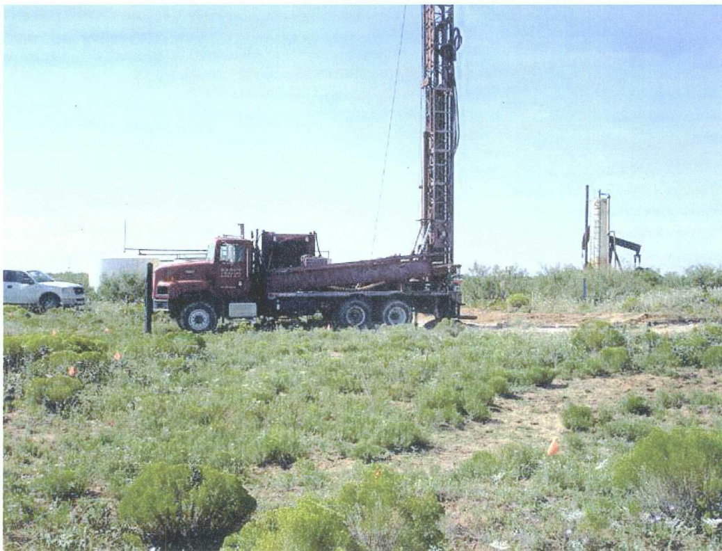
View facing southwest showing drilling of monitoring well MW-1 located adjacent to release point at the Santa Rita EOL Site. (08-30-05)
