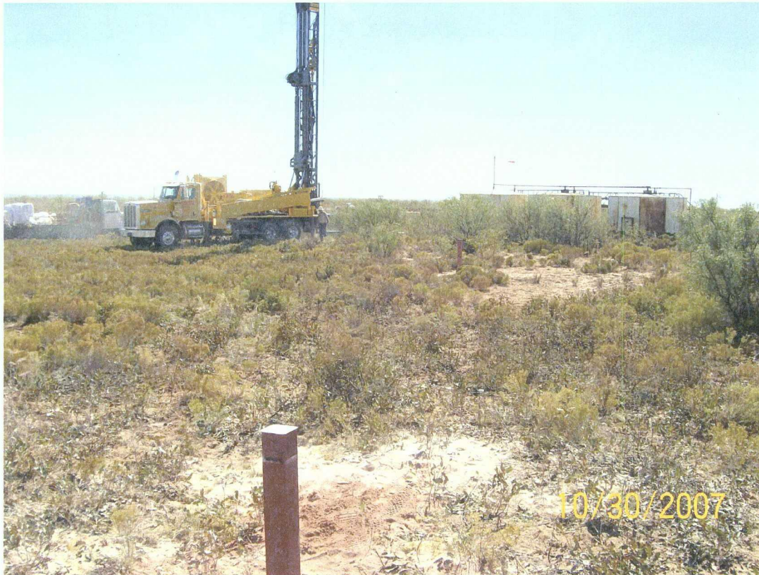
View facing southeast showing completed monitoring well MW-2 (foreground) and drilling rig at downgradient MW-3 (background)
