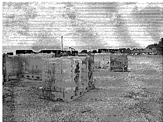
Photo 12: Tote tank located directly on ground.
