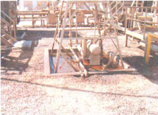
Photo 15: Fluids in another lube tank containment area.
