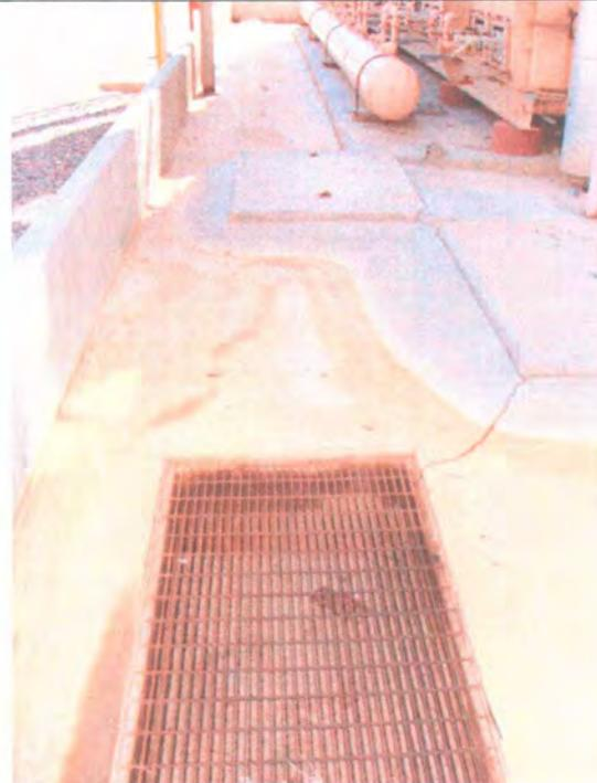
Photo 4: Sump in secondary containment of unused heater with a crack in containment.
