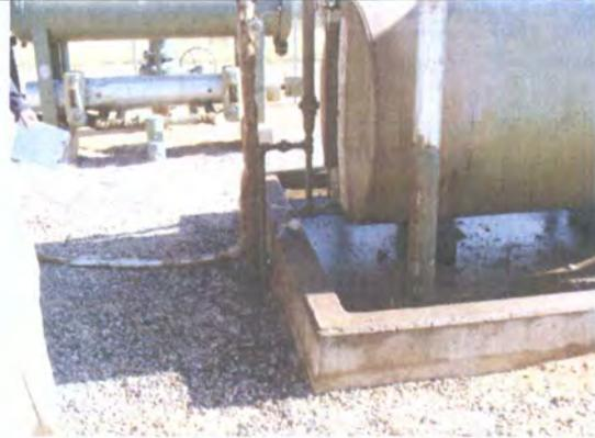
Photo 4: Stained soil near saddle tank.
