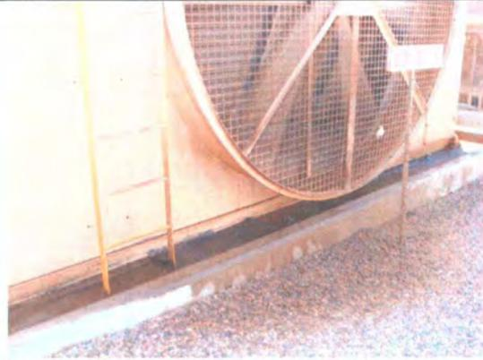
Photo 10: Gravel/soil staining near fan.
