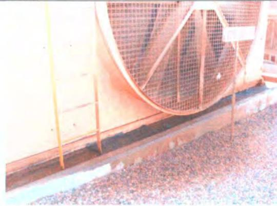
Photo 10: Gravel/soil staining near fan.
