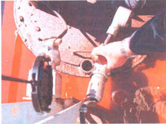
Photo 1: Leak detection in submerged sump.
