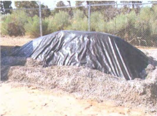
Photo 3: Contaminated soil covered in plastic.
