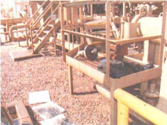
Photo 14: Gravel/soil staining near compressor engines.
