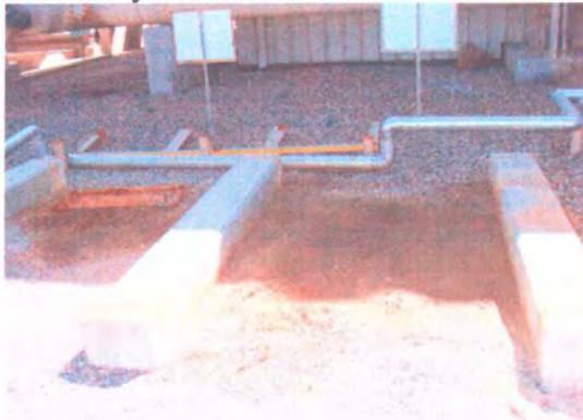
Photo 25: Soil staining on ground.
