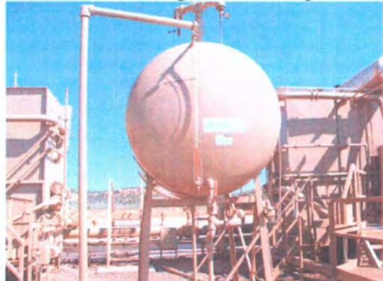
Photo 23: Label on tank is not legible.
