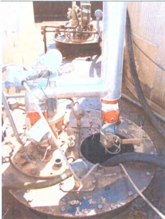
Photo 19: One of two sumps in secondary containment for used oil and condensate tanks.
