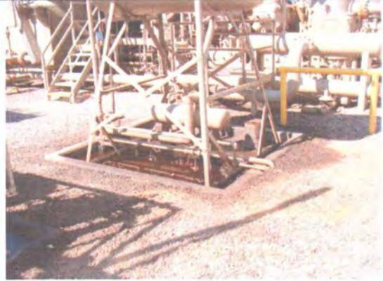
Photo 16: Staining around another lube tank area.
