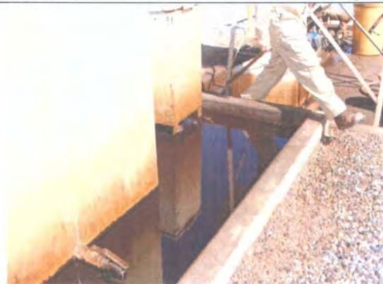
Photo 21: Standing fluids in secondary containment area.
