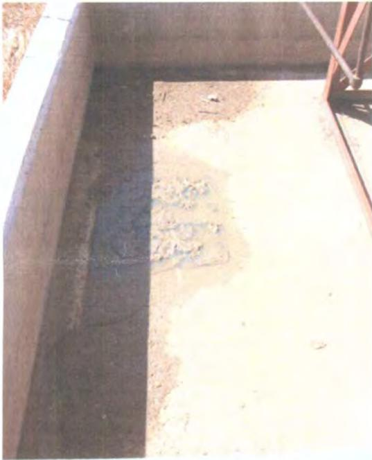
Photo 24: Standing fluid in methanol secondary containment area.
