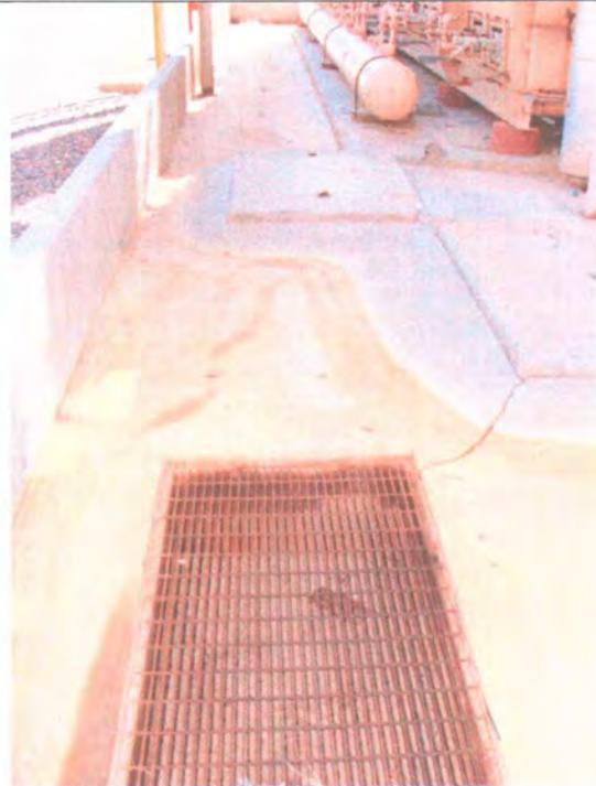
Photo 4: Sump in secondary containment of unused heater with a crack in containment.
