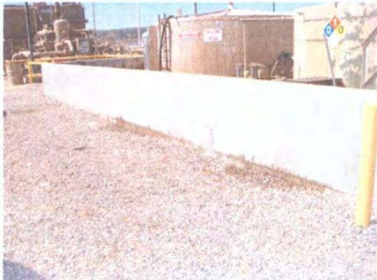
Photo 20: Secondary containment for Used Oil and Condensate tanks appear to be leaking.
