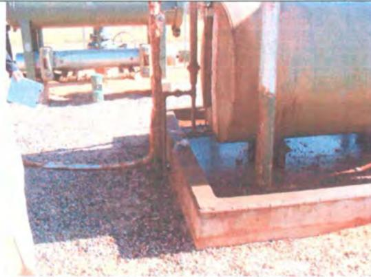
Photo 4: Stained soil near saddle tank.
