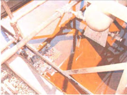
Photo 13: Saddle lube tank with fluids in secondary and a clogged drain.
