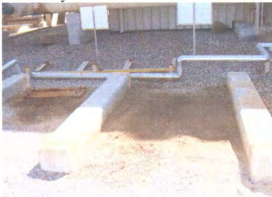
Photo 25: Soil staining on ground.
