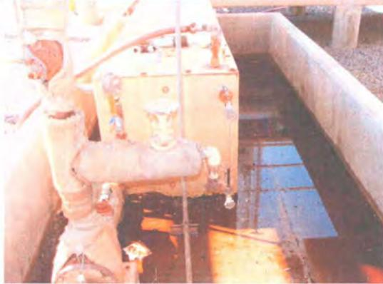
Photo 7: Fluids within secondary containment of amine recovery tank.
