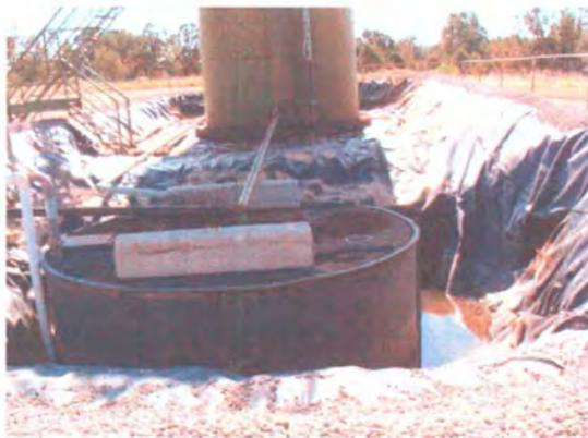
Photo 6: BGT has fluids/water in its bermed area.
