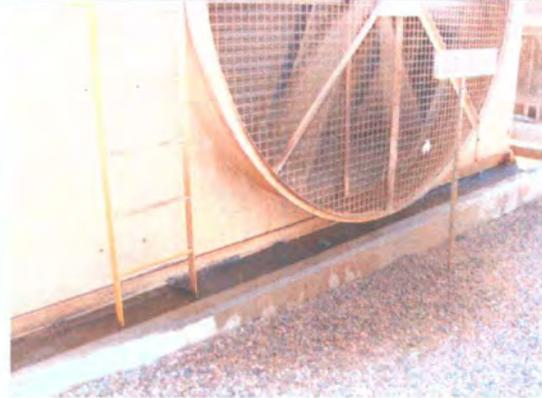
Photo 10: Gravel/soil staining near fan.
