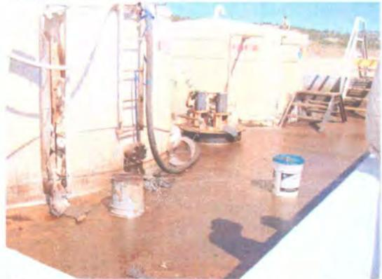
Photo 18: Secondary containment for used oil and condensate tank. Staining on floor.
