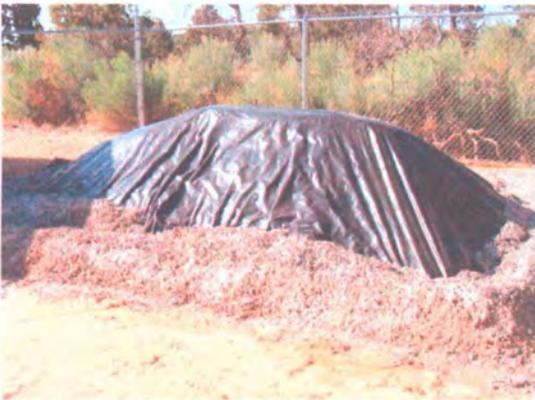
Photo 3: Contaminated soil covered in plastic.
