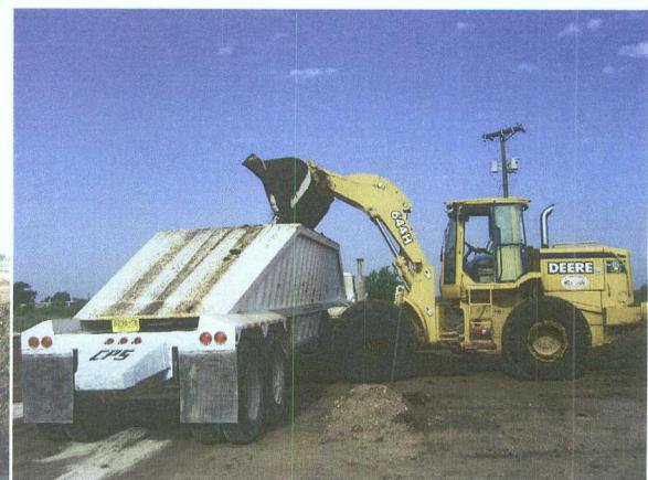
4. 51,000 cubic yards of clean backfill was transported, placed, and compacted.
