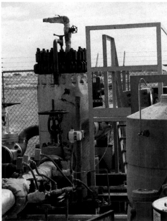
Filtration system before injection w/ boxes for O&M by workers
