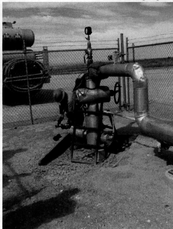
Wellhead w/ Hot Oil Operator preparing to install chart recorder for MIT
