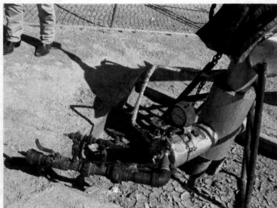
Connection to annulus through small 1/2 inch dia. fitting
