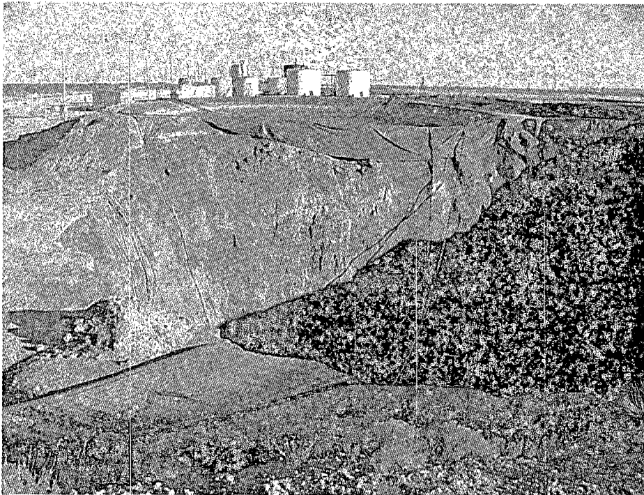
Loco Hills brine well collapse , morning, November 7, 2008, sinkhole with fresh water pond in foreground. Photo courtesy of Oil Conservation Division
