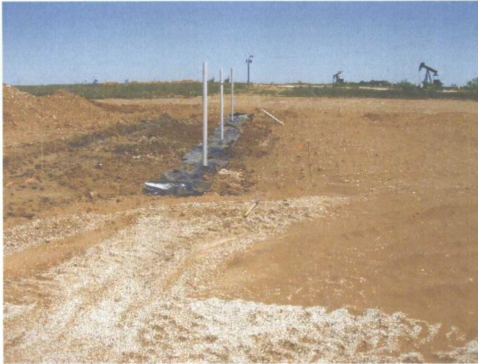
Soil Vapor Extraction System Installation Looking East
