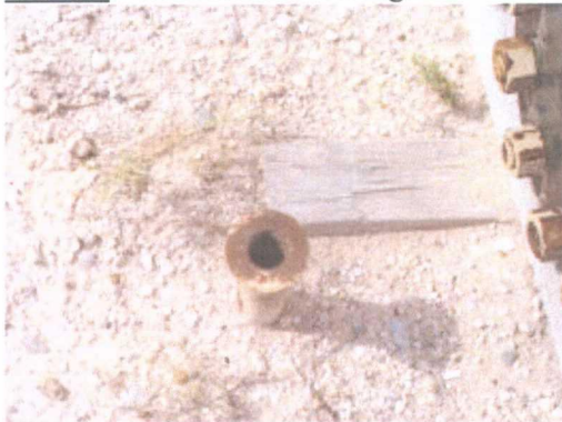
Photo 3 : Underground conduit protruding from ground level near concrete slab.
