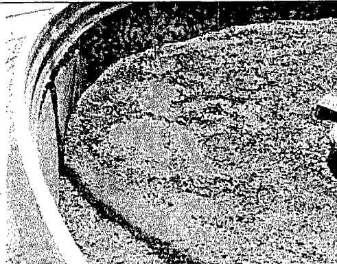
Photo 4 : Free liquids in secondary containment.
