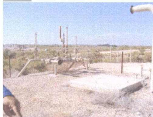
Photo 4 : Remaining concrete slabs with exposed conduits.
