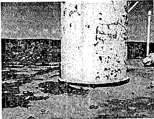
Photo 1: Used tank not in service. Leaking substance on to ground.
