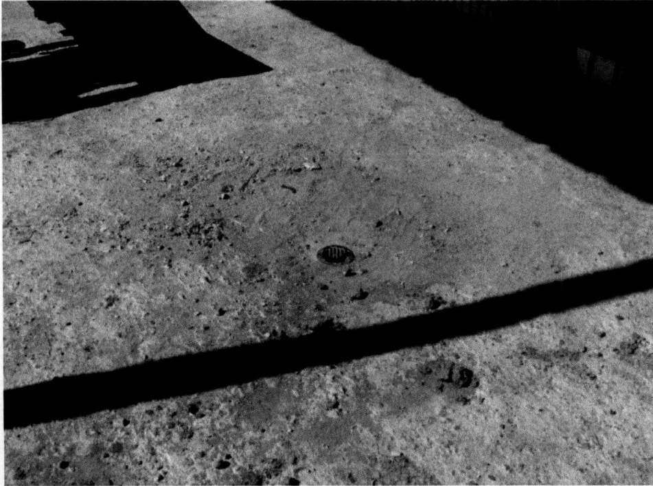
Photo 5: Drainage in chemical storage area. Cement containment is wearing and is porous.
