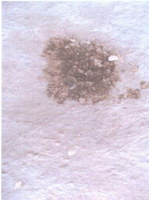
Photo 6: Drain in padded containment area. Drains to the south and outside of covered area.
