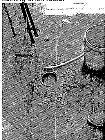
Underground Injection Control (UIC) EPA Class V Well where chemicals may leach into the Ogallala drinking water aquifer beneath the facility.
