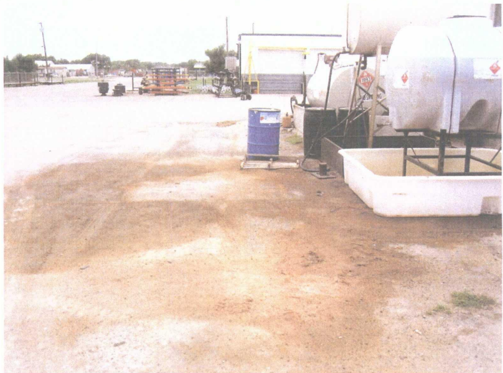
Photo 2 - View of hydrocarbon staining around AST containment area; pre-remediation
