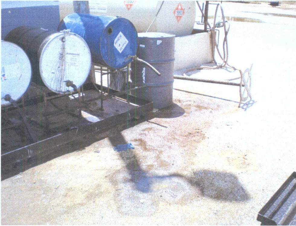
Photo 1 - Before; chain oil leaking from spout/hose
