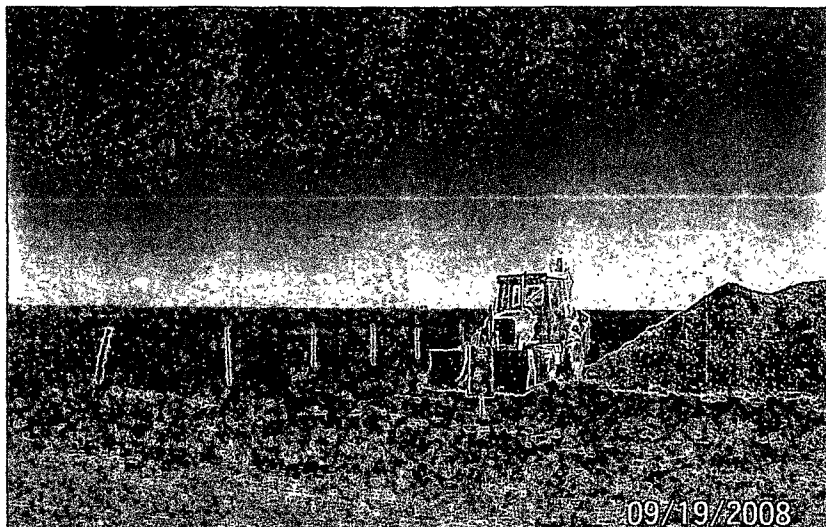
Photo #21 Digging out Impacted Soil
