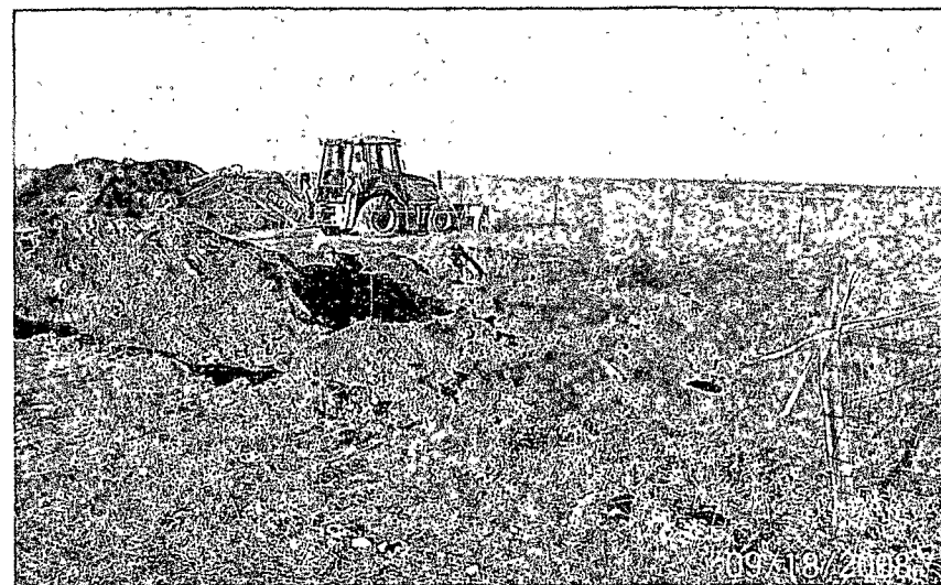
Photo #18 Digging out Impacted Soil
