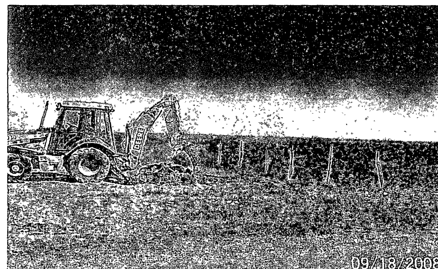
Photo #12 Digging out Impact Soil
