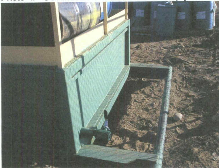
Photo 5. Valve to Drain Containment Bin for Empty Drums
