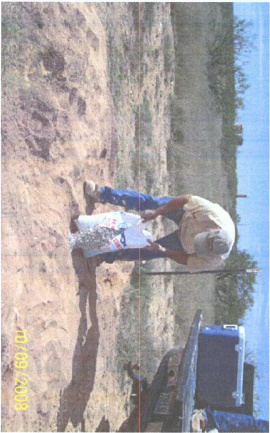
Plugging SB #1 with bentonite 2 days later
