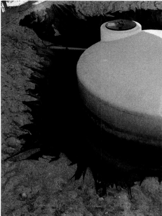
Photo 2: Unidentified poly BGT, single walled with liner.
