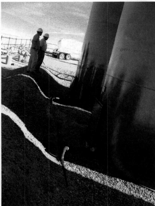
Photo 1: 3 AST's bermed, no liner.
