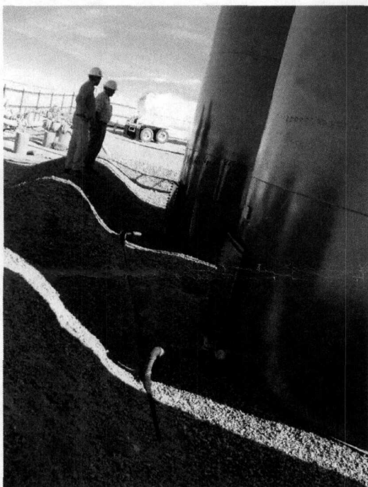
Photo 1: 3 AST's bermed, no liner.
