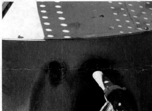
Photo 9: Evidence of overflow from 2 below-grade tank.
