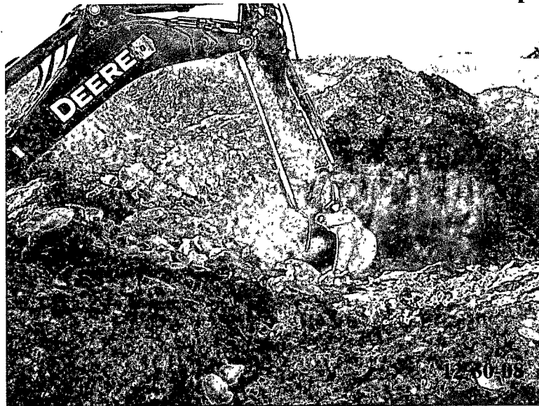
Excavation of impacted soil below workover pit.
