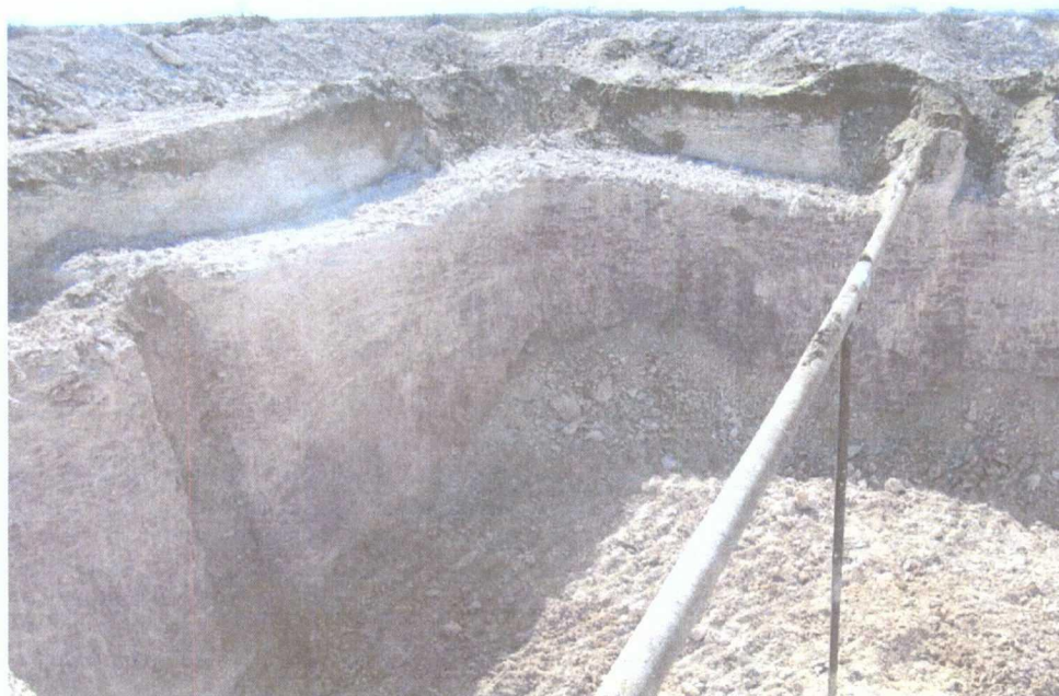
DCP Plant to Lea Station 6-Inch #2 release site excavation
