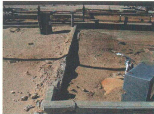
Photo 5: Breached secondary containment wall.
