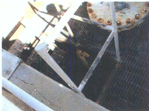
Photo 8: BGT with cracked containment.
