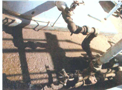
Photo 12: Sediment and hydrocarbon staining in secondary containment area.
