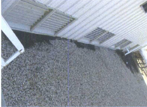
Photo 35: Hydrocarbon waste breaching the compressor building.
