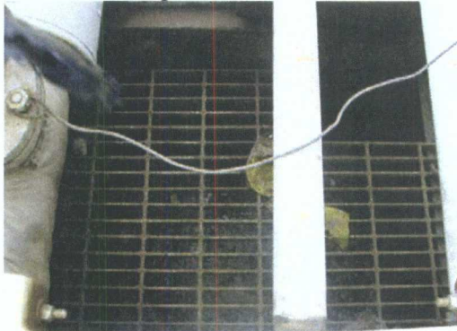
Photo 2: Debris in sump.
