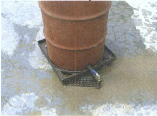
Photo 3: Sump full of sediments.
