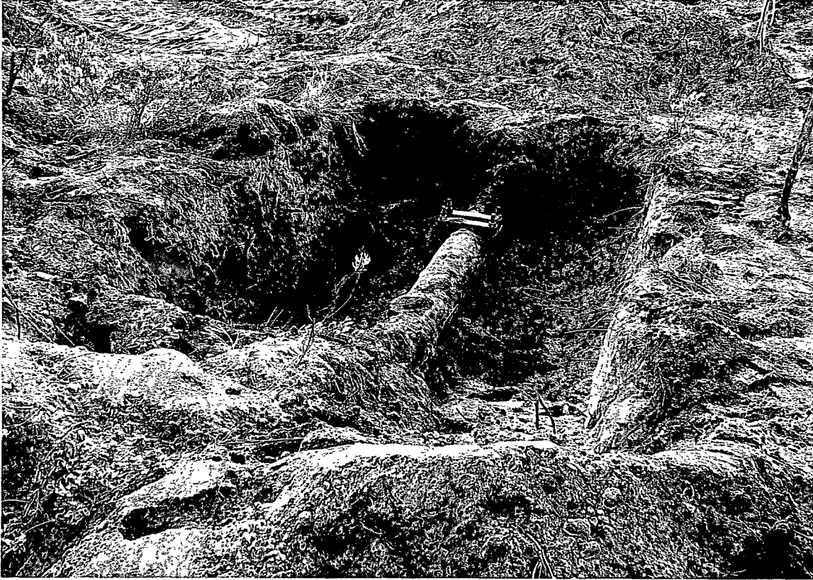
Initial excavation and clamp on line
