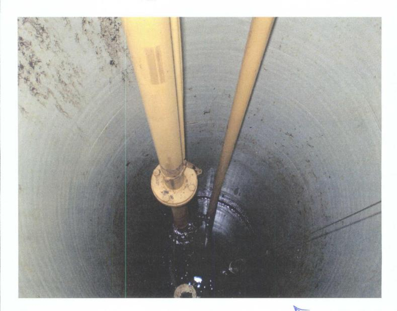
2009 Gallup Station Oily Waste Water Sump by Engine Room This is a fiberglass sump with auto dump controls Swaby MFG Co.
