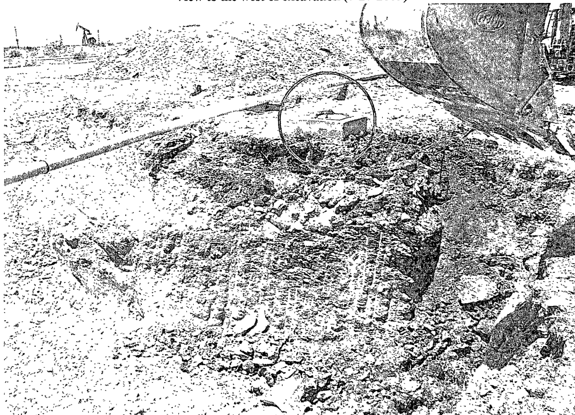
Northwest sidewall of excavation and surface completion of out of service water supply well? (7-27-2009)
