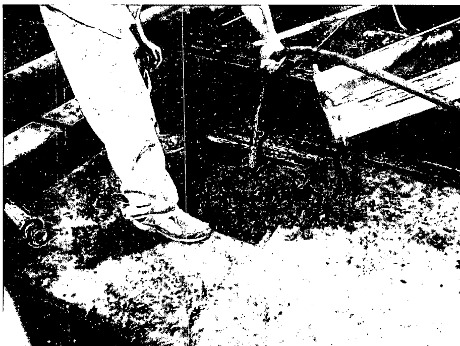
The cementing of the Wash Bay sump.
