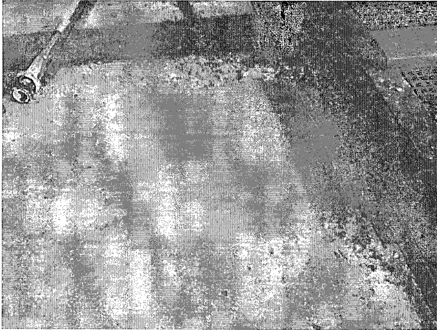
View of former Wash Bay sump filled with cement.
