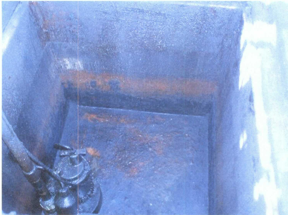
View of sump, transfer line, and pump in the secondary containment.
