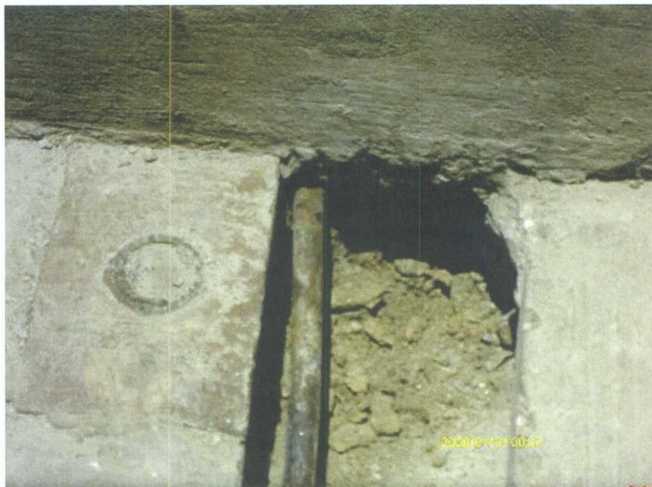
View of discolored soil and rusting pipe at the secondary containment sidewall.
