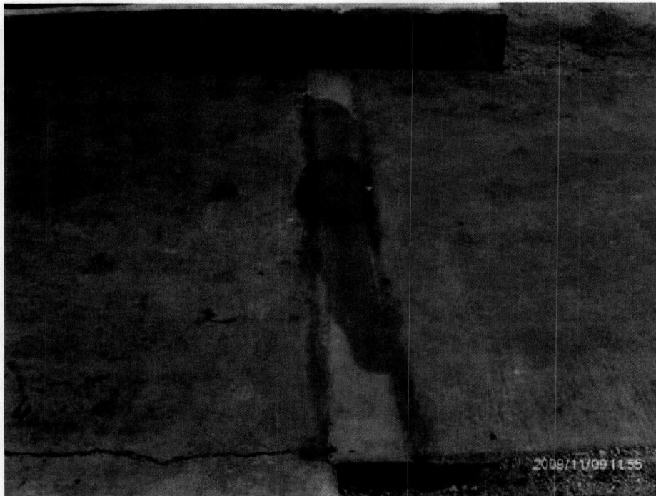
View of cement filled trench.
