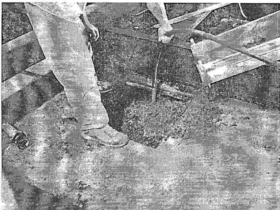
The cementing of the Wash Bay sump.
