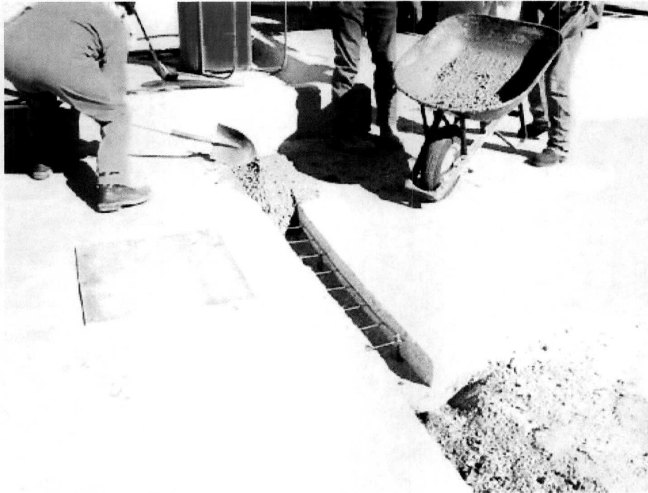
View of trench being filled with cement.
