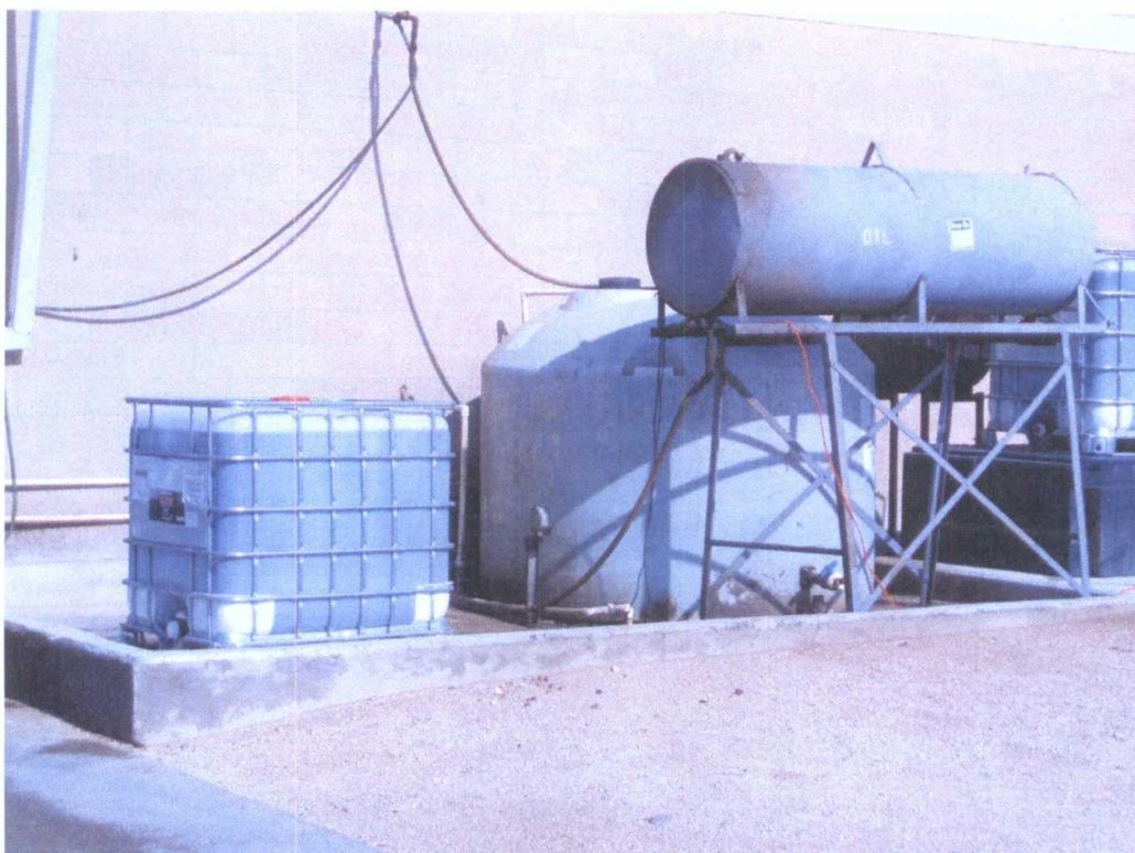
Viewing north of secondary containment with Mop Wash Water Tank.
