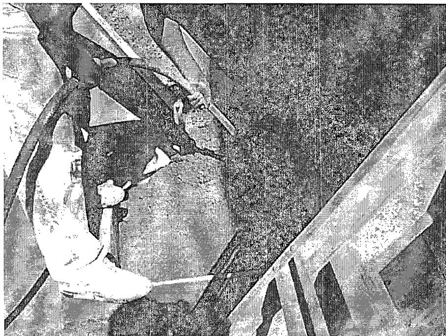
Another view of the South Drain sump being filled with cement.
