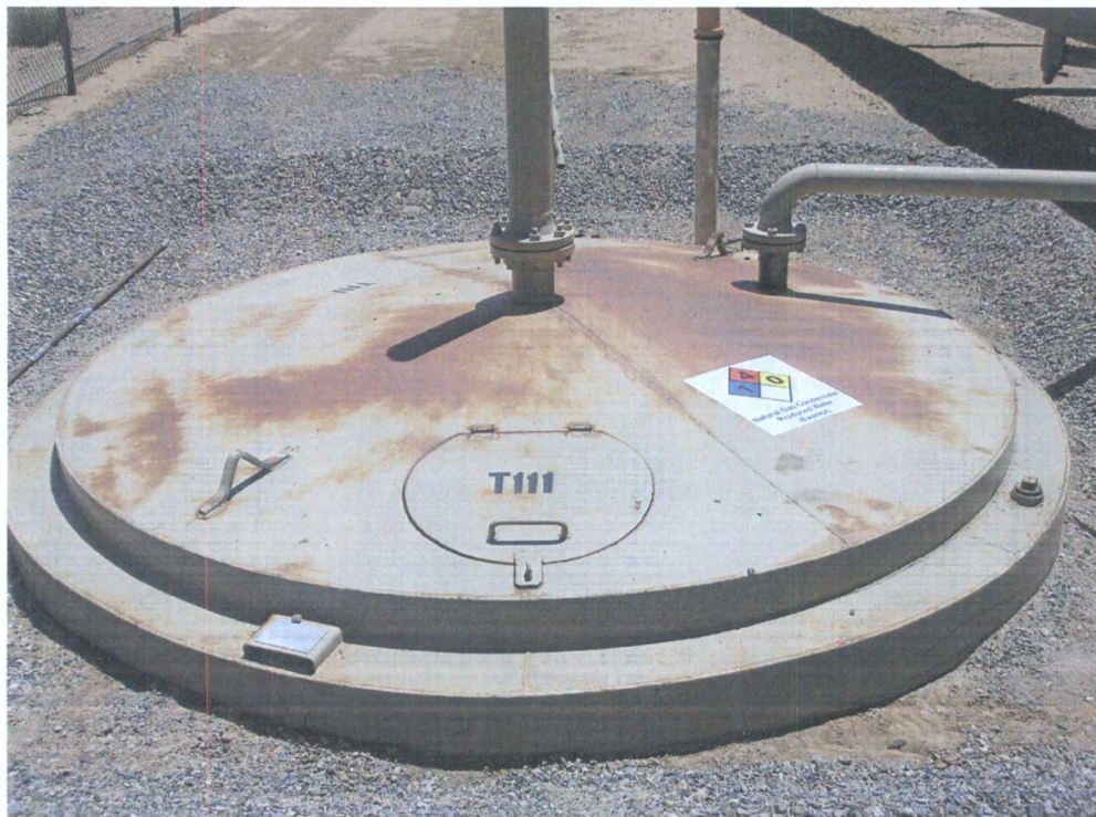
Sub-Grade drain tank used to capture condensate/produced (exempt) water from pigging operations with label.
