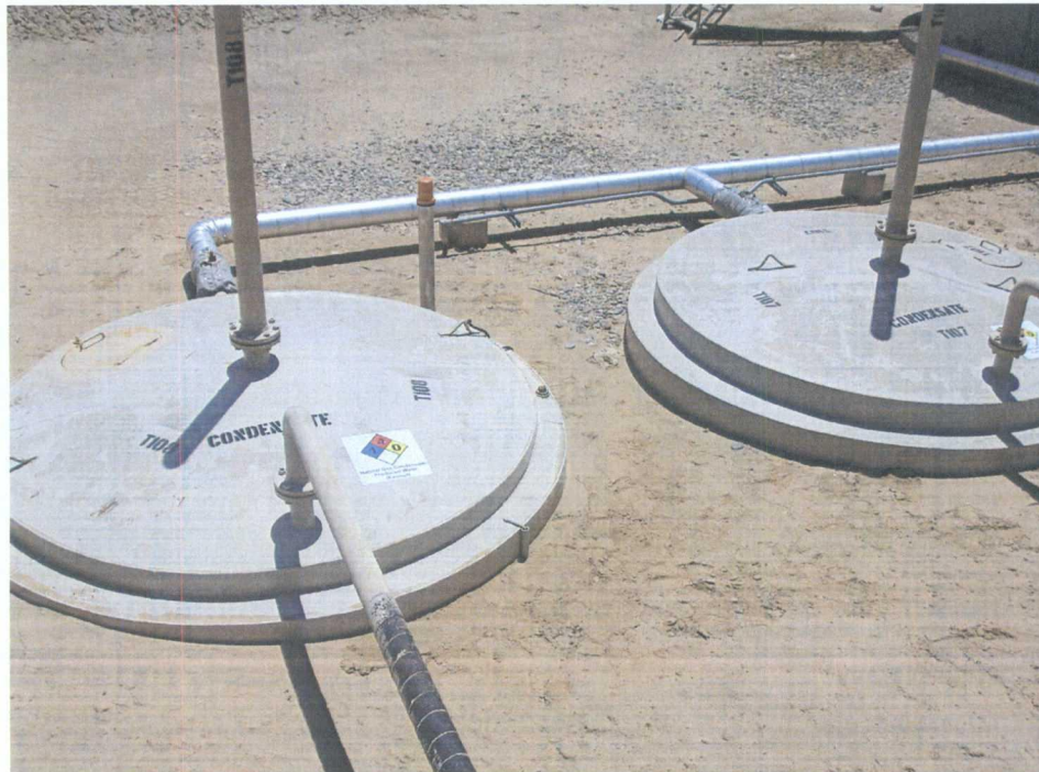
Sub-Drain Tanks labeled "Condensate" with NFPA Diamond.
