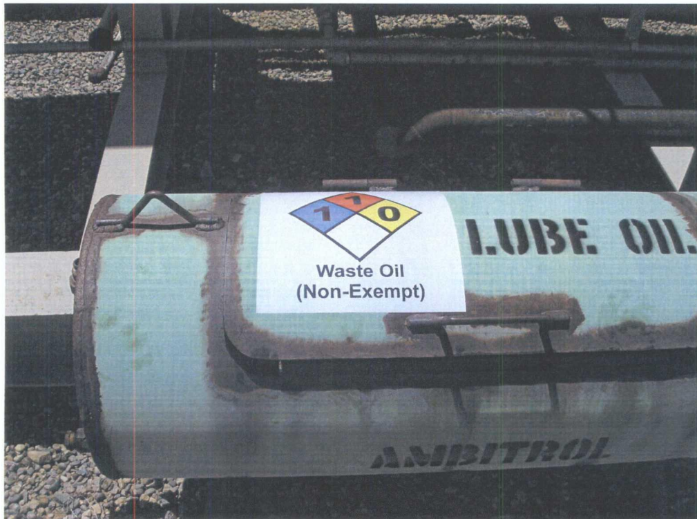
Small container used to drain filters and for temporary storage of used oil
