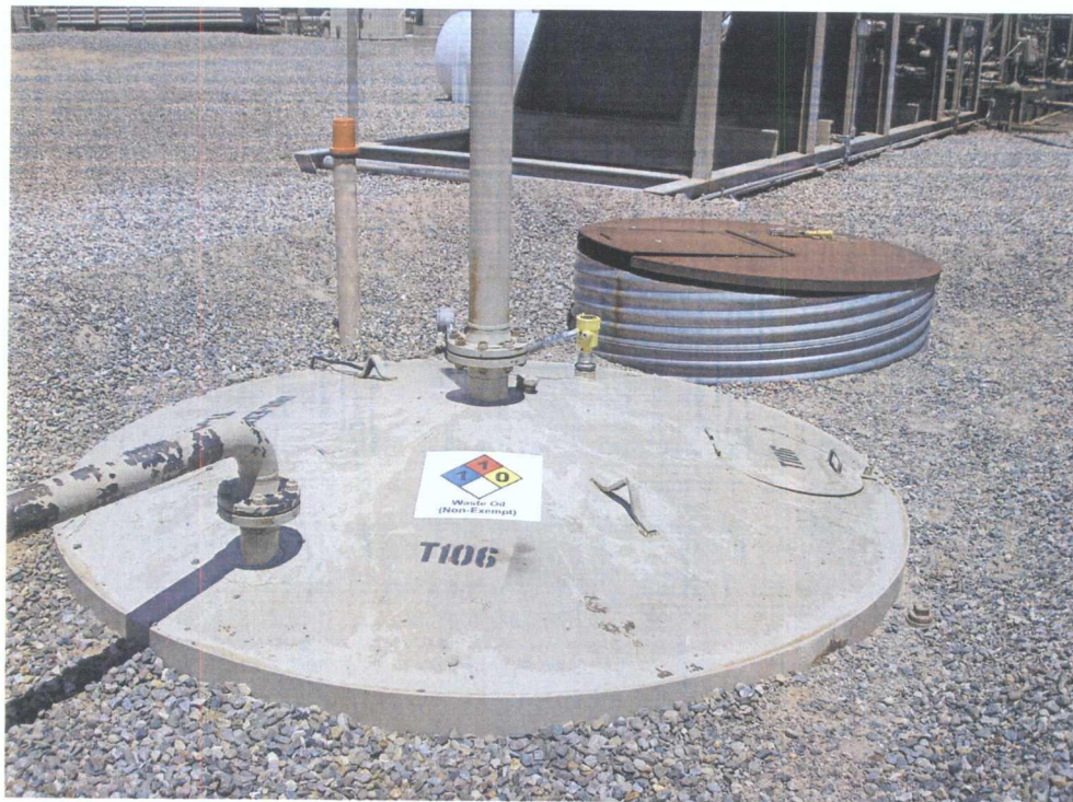
Sub-Grade Waste Oil Tank (Non-Exempt) with label.
