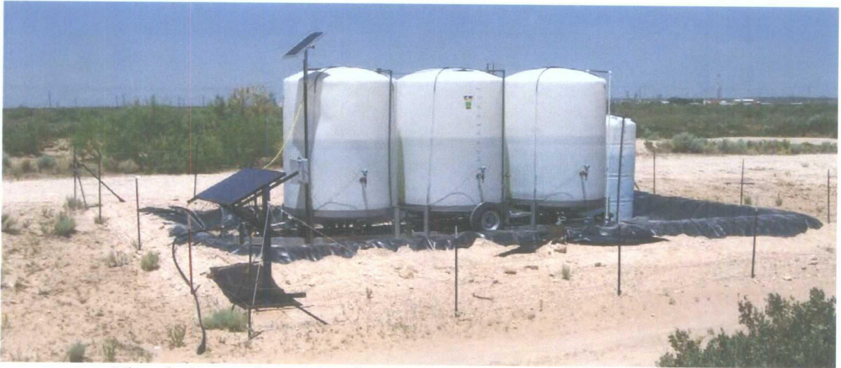
View facing northwest showing groundwater recovery system at RW-1
