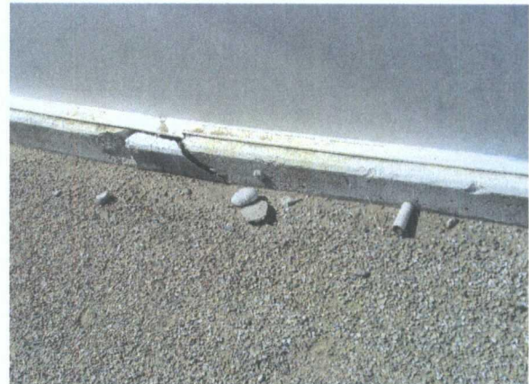
Tank 815 Perimeter concrete ring fracture w/ pigtail drain @ 90° angles
