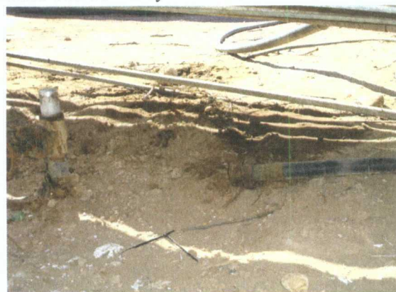
Small leak in one of the Carbon Black Oil lines beside slurry oil treatment area
