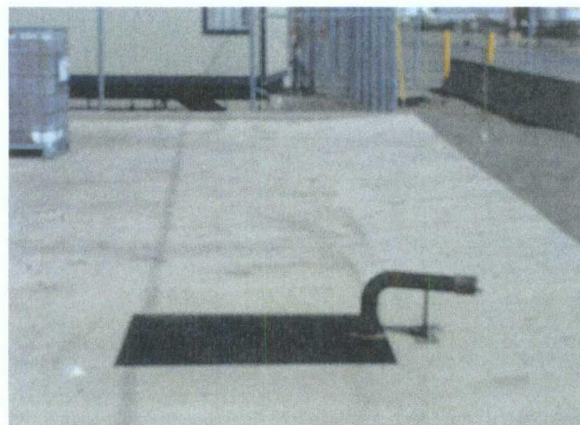
Central chemical storage sump w/ leak detection system
