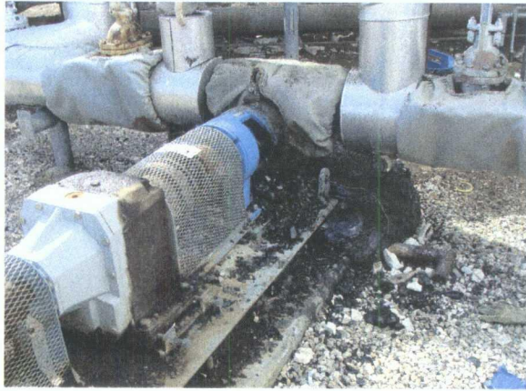
Pitch tar piping leak evident
