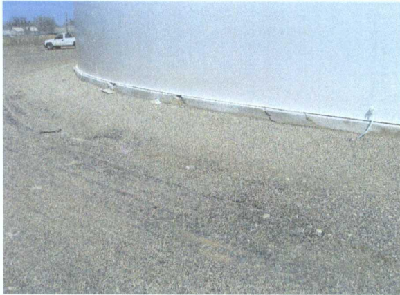
Tank 815 Perimeter concrete ring
