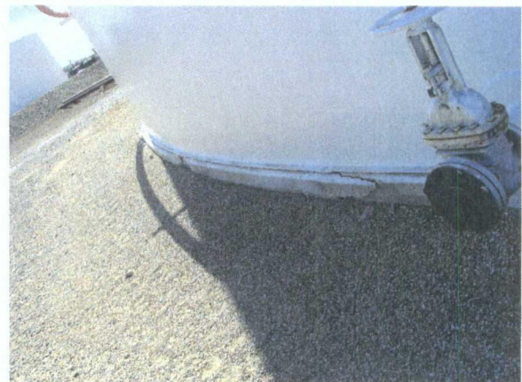
Tank 815 Fractured concrete ring base
