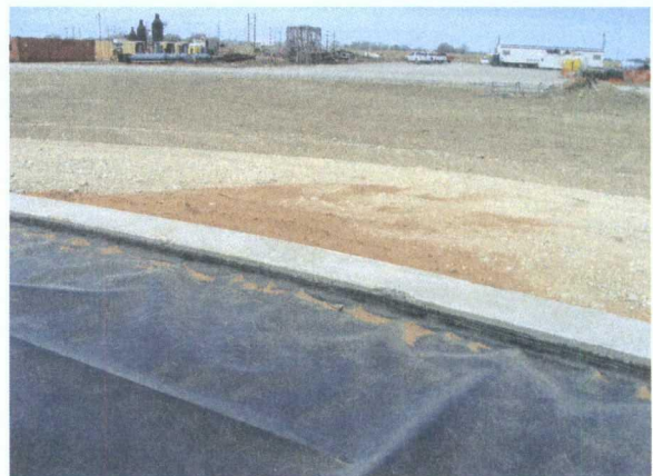
Tank 1225 Thermal welded liner to inner perimeter of concrete base ring
