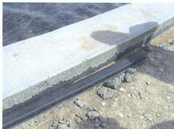
Tank 437 liner appears to be sandwiched into the top of concrete base ring
