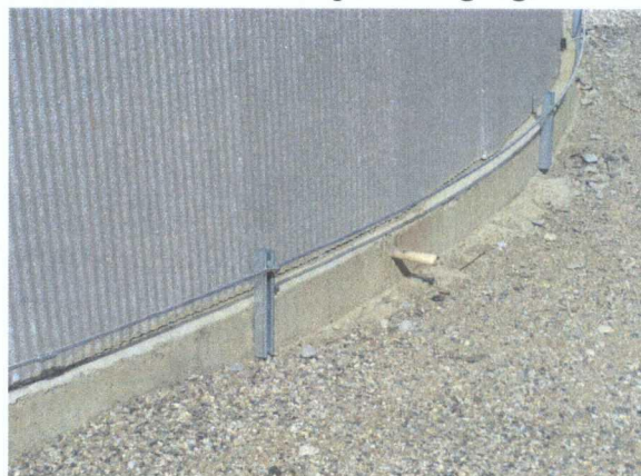
Pitch Tank 814 concrete base ring w/ pig tail design and high temp liner
