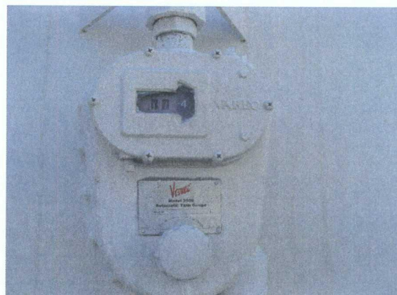
Tank 815 Fluid Level Indicator reading 17.4 ft. of fluid in tank
