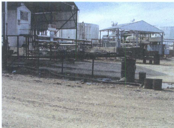
New Rose Unit installed at the former Tank 437 area to treat heavier Canadian Crude (~18K bbl/day)
