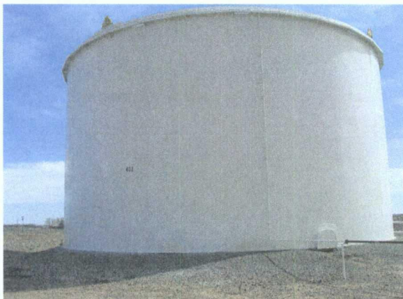
Tank 402 constructed on ground w/o concrete base ring construction, liner & pig tail drainage system
