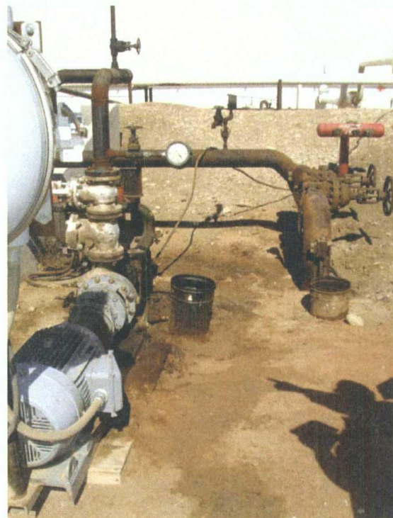
Contamination on ground from leaky crude oil transfer pump in need of cleanup & secondary containment.
