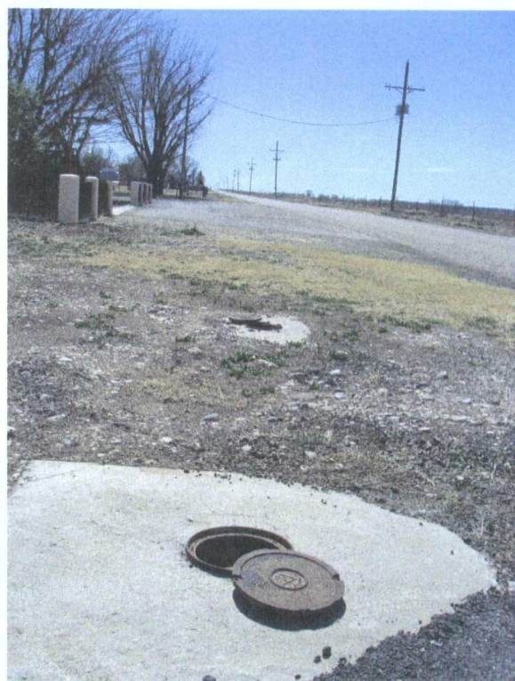
Looking S along S. Bolton Rd. at flush mount MWs E of roadway- wells unlocked
