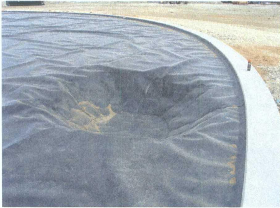
Tank 437 Sump area ~ 5ft x 7 ft some pressure loss noted on E side thought to be heat related (Matrix Services, Inc. John Dyring 282-458-8781)
