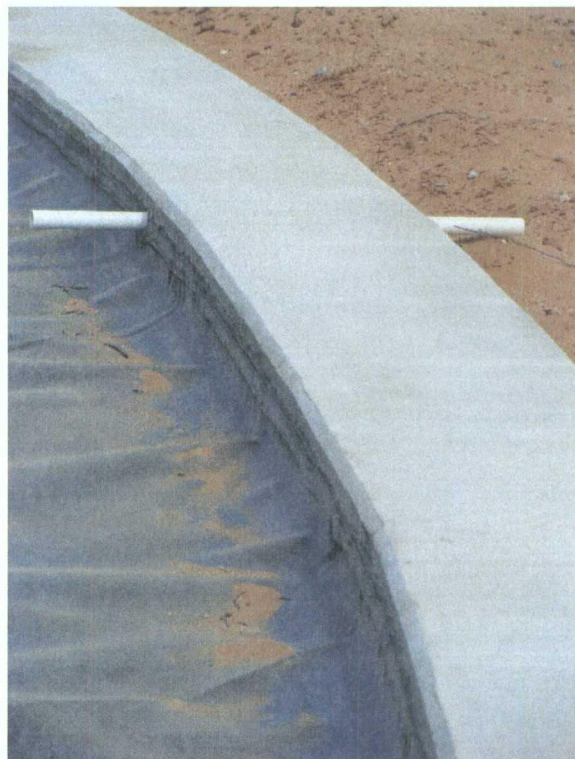
Tank 437 One inch tattle tale leak detection system pipe oriented at 90° angles
