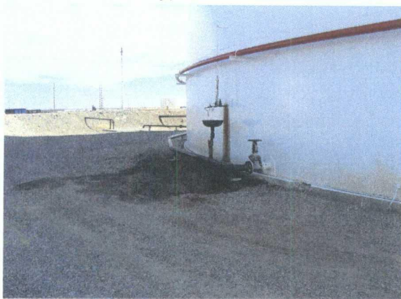
Tank 815 (80K bbl) Built ~ 2 yrs. ago. Ultra-low sulfur diesel leak needs cleanup and investigation to determine if fractured ring base has caused a leak in the tank?
