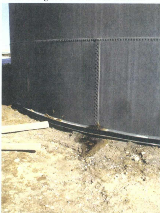
Tank# 59 CBO leak
