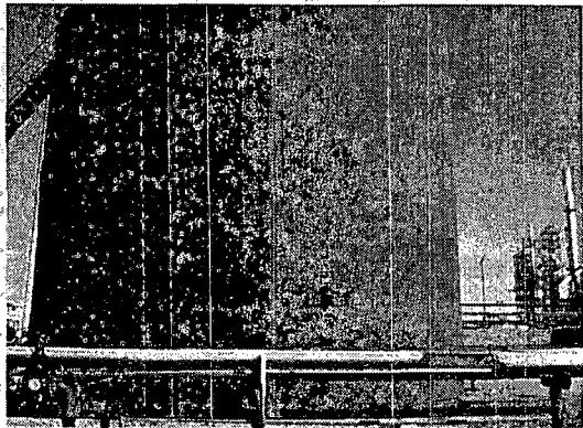
Tank# 58 signs of CBO leaks
