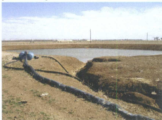
Line w/ pump to use fresh water in storm water retention pond when necessary.
