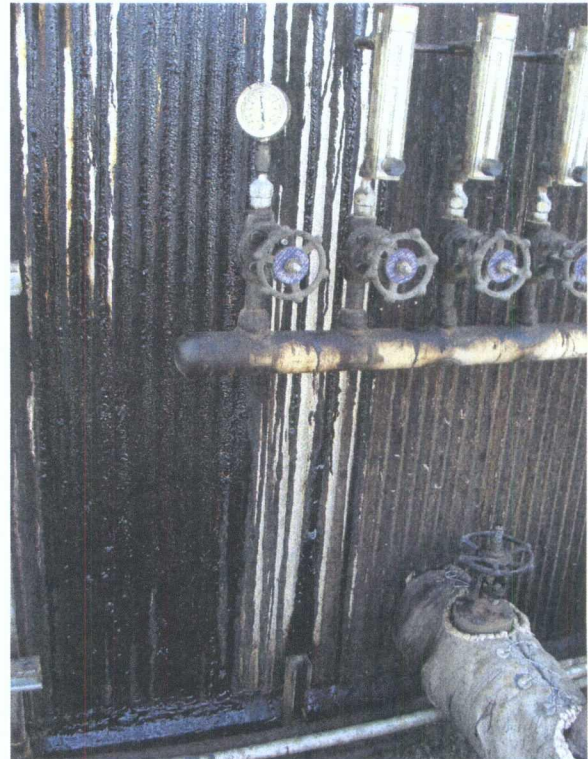
Pitch Tank 814 Close up on tank gauging station
