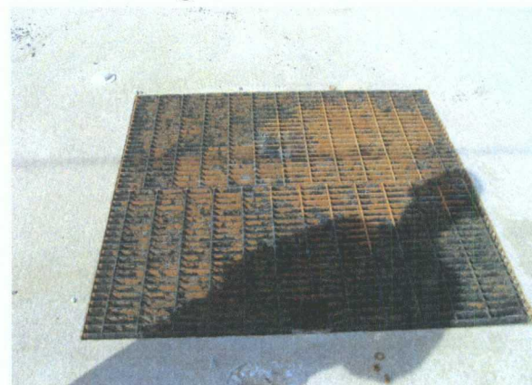
Close-up of sump w/ leak detection system location on pad in central chemical storage area
