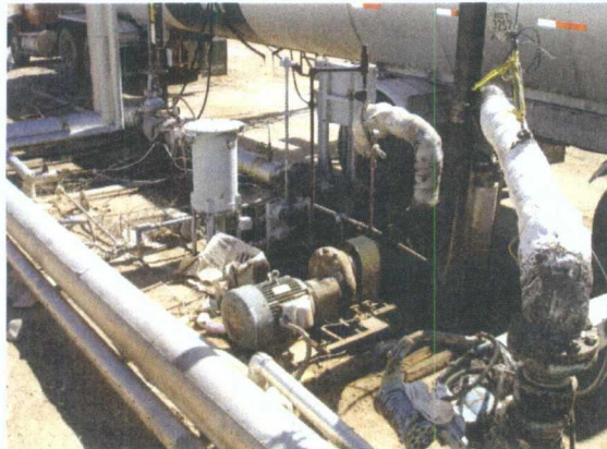
Issue 6- gas-oil pumps sump - area not in service
