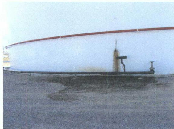
Tank 815 low-sulfur diesel leak from water withdrawal location
