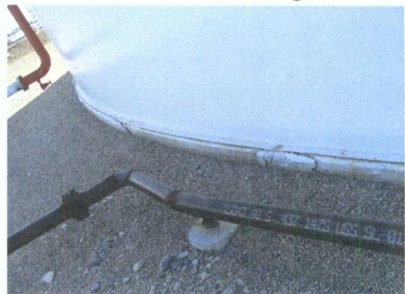
Tank 815 Fractured concrete ring base
