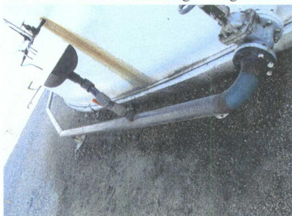
Tank 815 water draw leak location close-up
