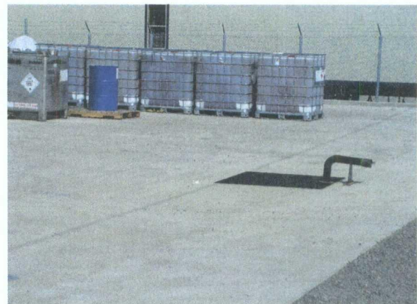
Central chemical storage pad w/ drainage sump location to control spills
