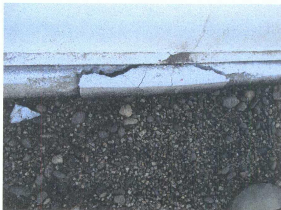
Tank 815 Concrete ring break (tank installed off-center) & w/o liner underneath, but w/ pigtail drains
