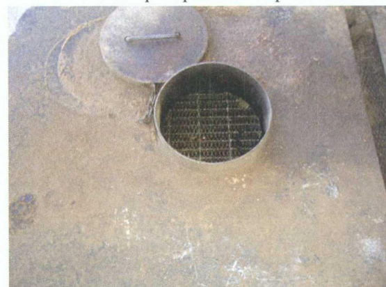
South Gasoline pump area sump
