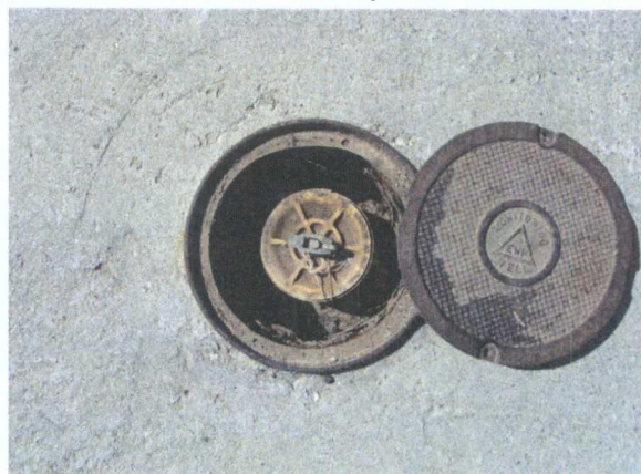
S Bolton Rd. flush mount MW at recovery well area to stop migration of GW contamination from moving further SE
