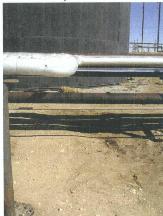
Small leak in carbon black oil line beside Tank# 58
