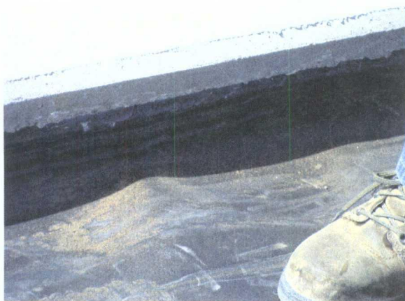
Thermally welded seam against concrete ring
