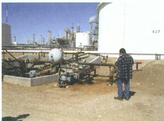
Crude oil pump area near Tank 437 and LACT area- secondary containment not provided for all pumps, but needed badly
