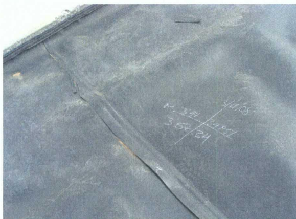
Tank 437 double weld seams w/ pressure test results in white chalk
