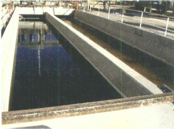
WWTP API used as settling basin for FCC fines
