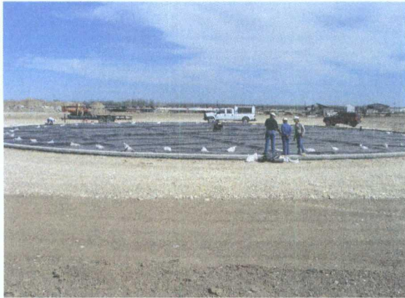
New Tank 1225 Crude tank (100K bbls) construction of concrete base ring w/ sub- liner (~120 ft. Dia.)
