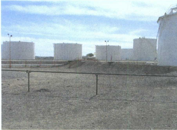
Older tanks constructed on top of ground w/o liner or concrete base ring design
