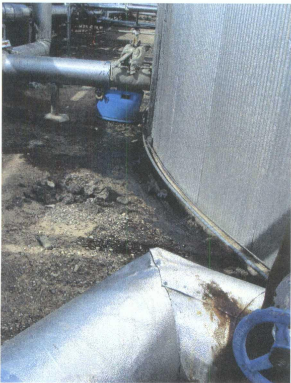
Pitch Tank 814 Investigate leaking bottom?
