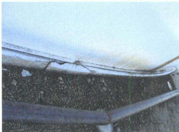
Tank 815 Concrete base ring fracture
