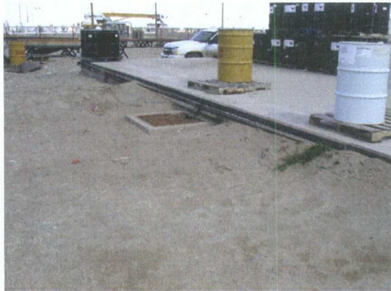
WH 5 drum storage pad catchment system full of sand w/ berm needed for containment
