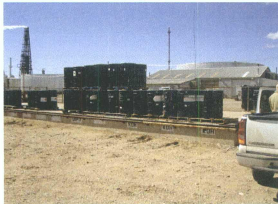
WH 5 Chemical drum storage pad-improper secondary containment
