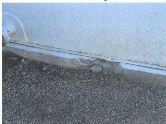
Tank 815 Concrete base ring damage
