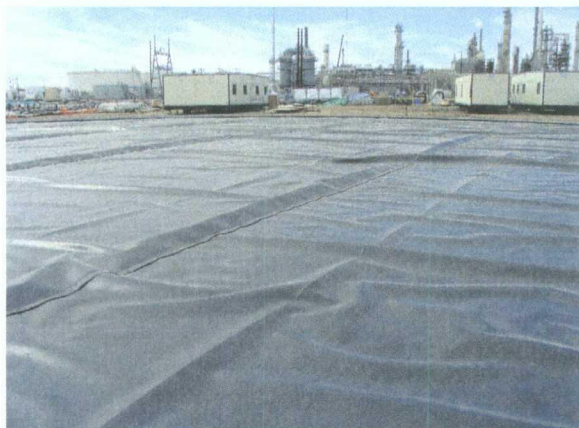
New Tank 437 location w/ 60-mil HDPE liner N of Tank 450
