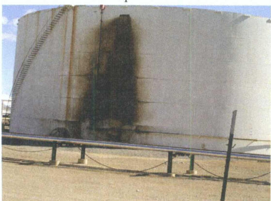
Tank# 439 release form tank due to overflow
