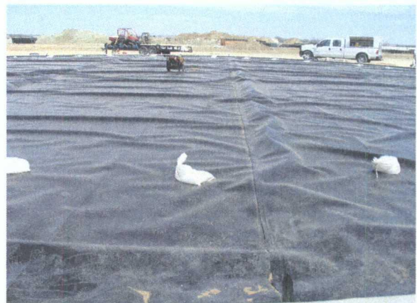
Tank 437 60-mil HDPE liner double seamed
