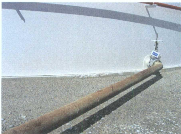
Tank 815 Fractured concrete ring base
