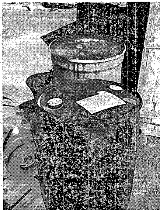
Improper storage of totes (no 2nd containment) WWTP
