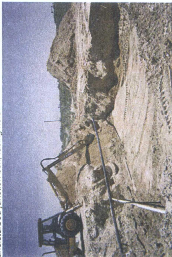
extending shelf, preparing for clay barrier
