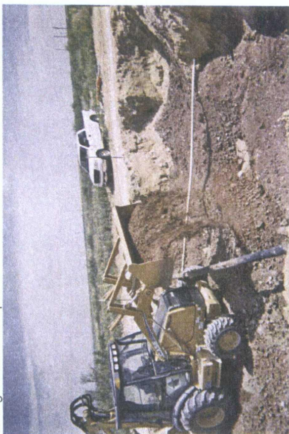
installing clay barrier
