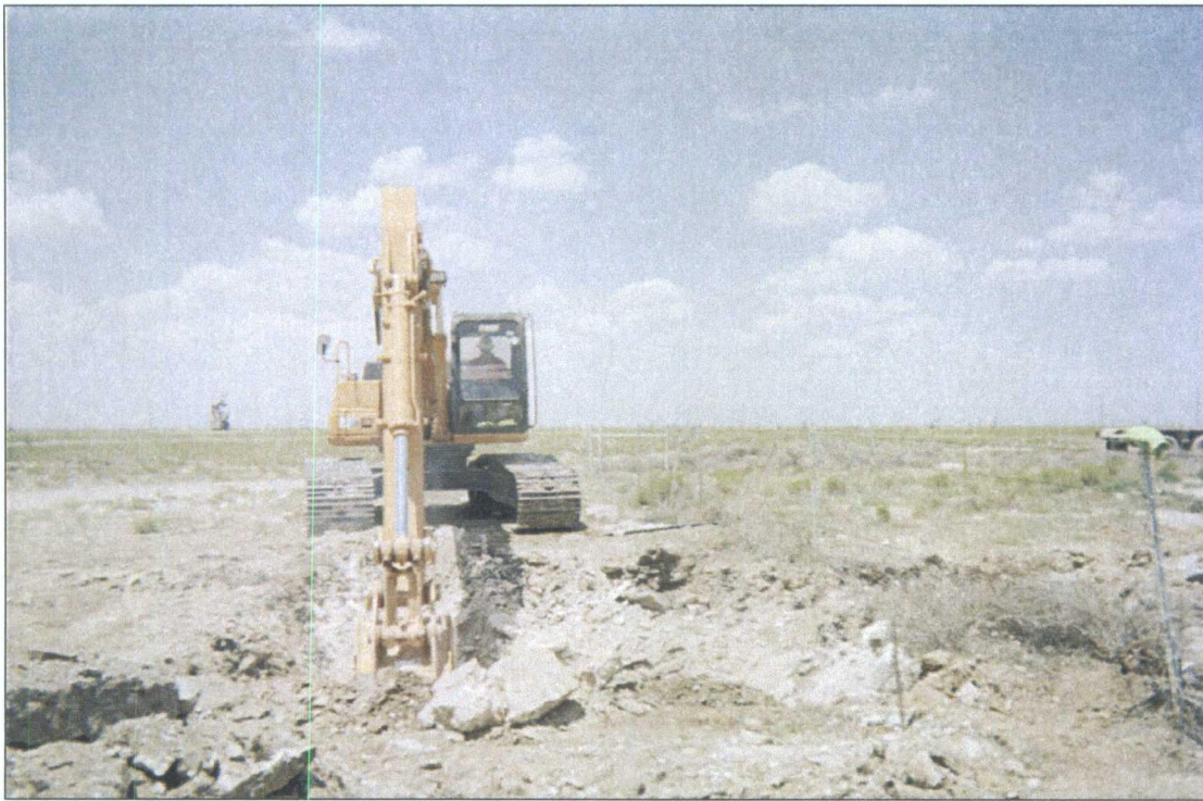
Figure 2 - Excavation of former junction box.
