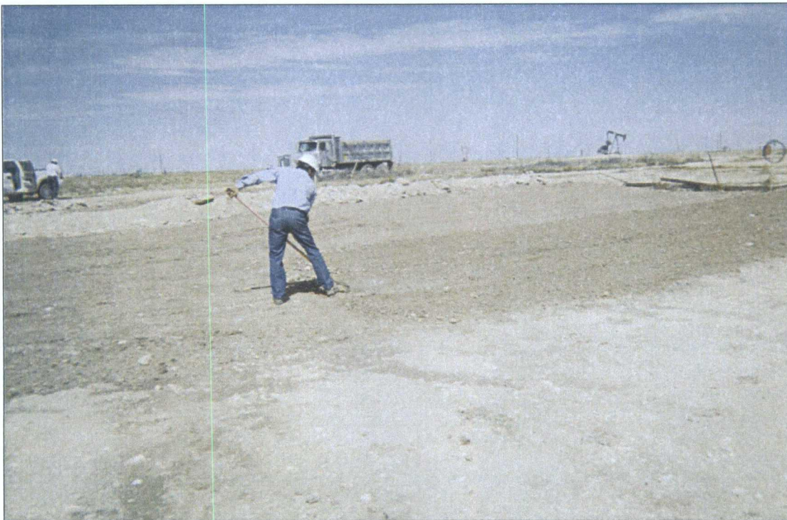
Figure 5 – Preparing the surface and reseeding with native vegetation mix.
