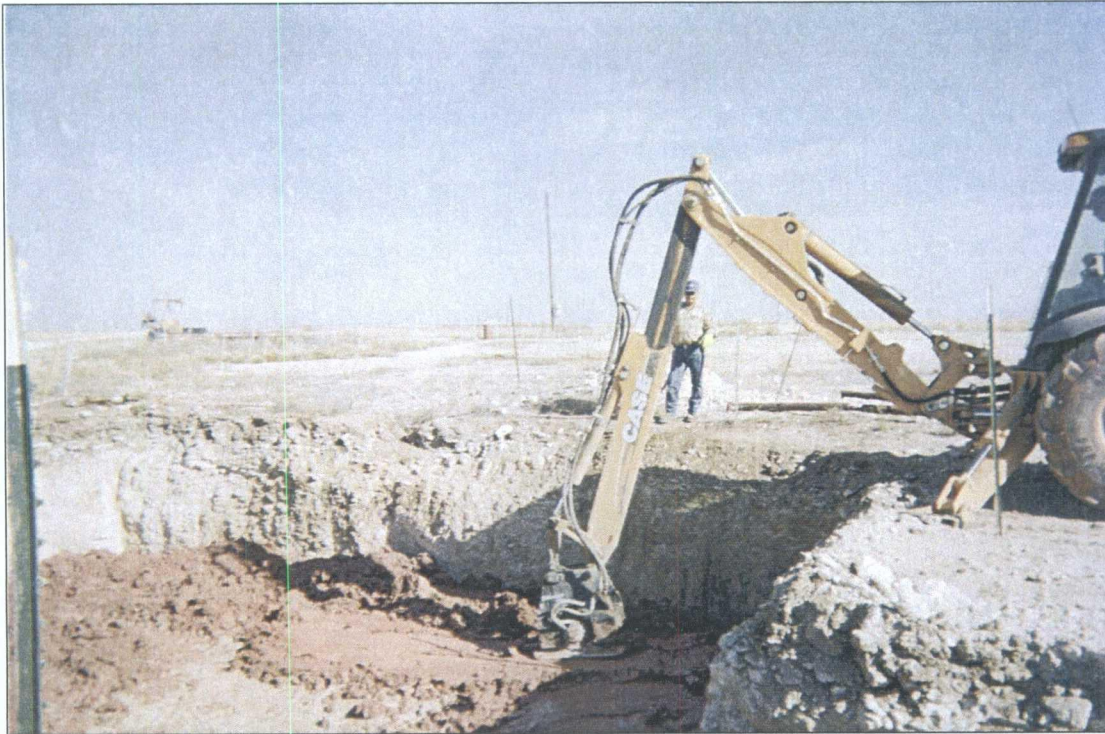
Figure 4 – Installation and compaction of sub-surface clay layer (infiltration barrier).
