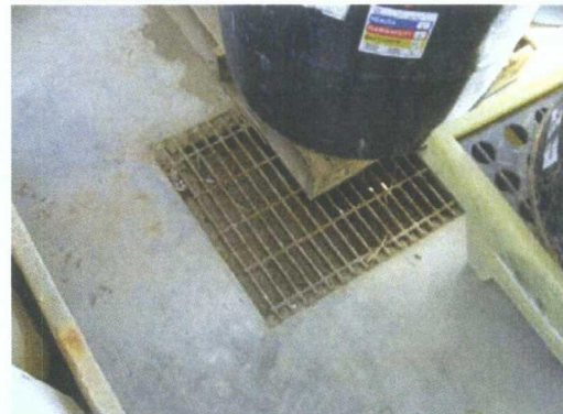
Photo 6: Sump in secondary containment.
