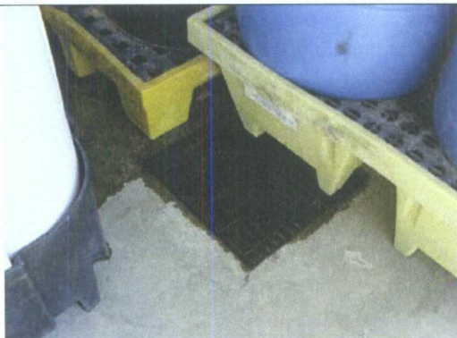
Photo 7: Sump with liquids in secondary containment.
