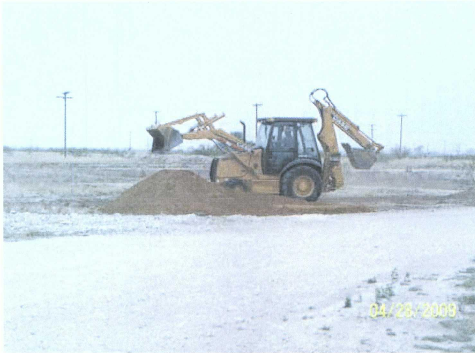
IMPORTING AND SPREADING SOIL
