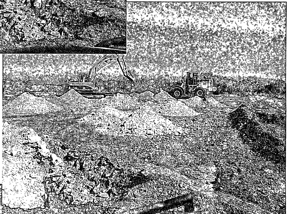
11/12/08 –Delineation of the release area with ten 4-ft trenches. >
