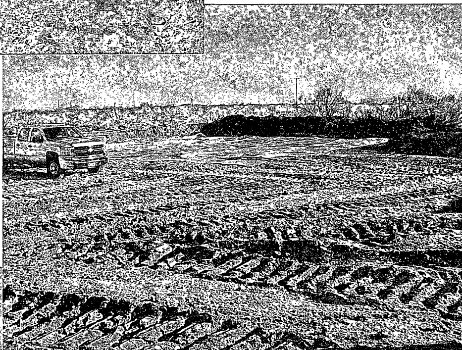
11/15/08 – Installation of 60' X 96' 20-mil liner. >
