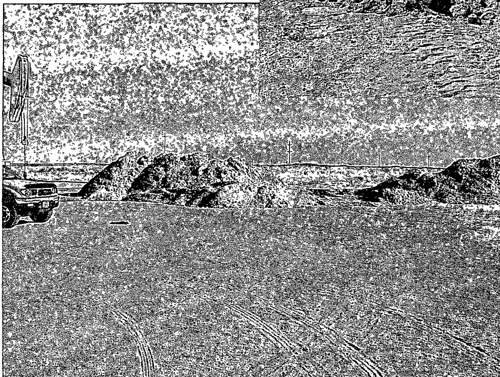
< 2/26/08 – Soil stockpiled on pad surface for blending
