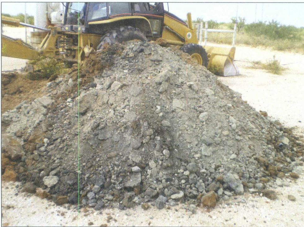
Figure 4 – View soil from bottom of sampling trench showing oil contaminated soil.
