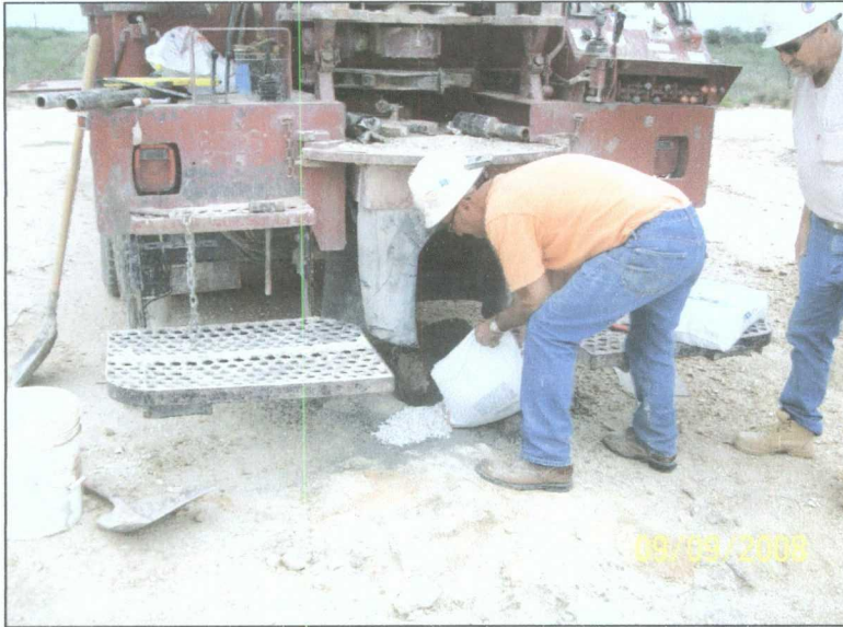
Appendix C – Harrison and Cooper plugging SB-1 with bentonite after completion of drilling.
