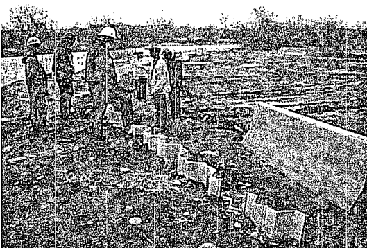
Pic22- Sheet piling and slurry wall installed next to the San Juan River to prevent hydrocarbons from seeping into river. Sheet piling is 11 feet deep, original design was to be 22 feet deep. Looking NE. upstream.
