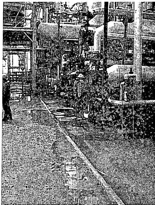
Pic9- Cat cracker area looking south. Picture shows pad and curb typical of all plant process areas.
