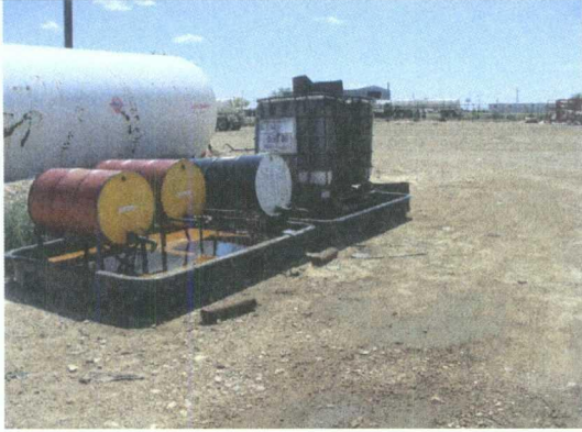
Photo 24: Secondary containments full of fluids. Staining on ground.
