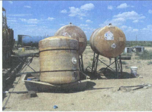
Photo 21: Improper location of saddle tanks.
