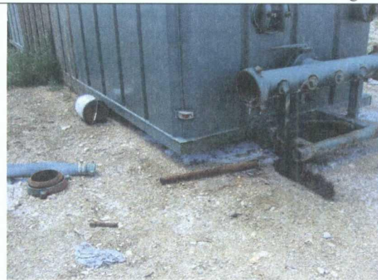
Photo 10: White residual staining near tank.
