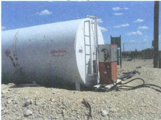
Photo 25: Improper lining of diesel tank.
