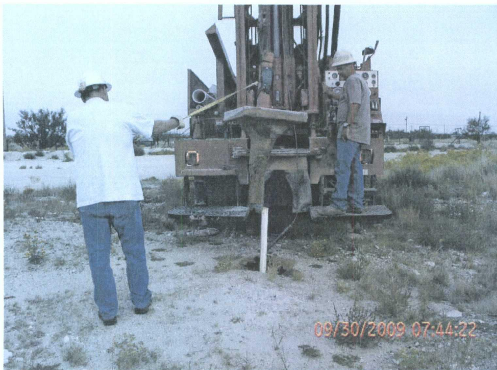
Plugging Well MW-1 at Hobbs B-32 Boot, NMOCD Case #1R428-57 9-30-09
