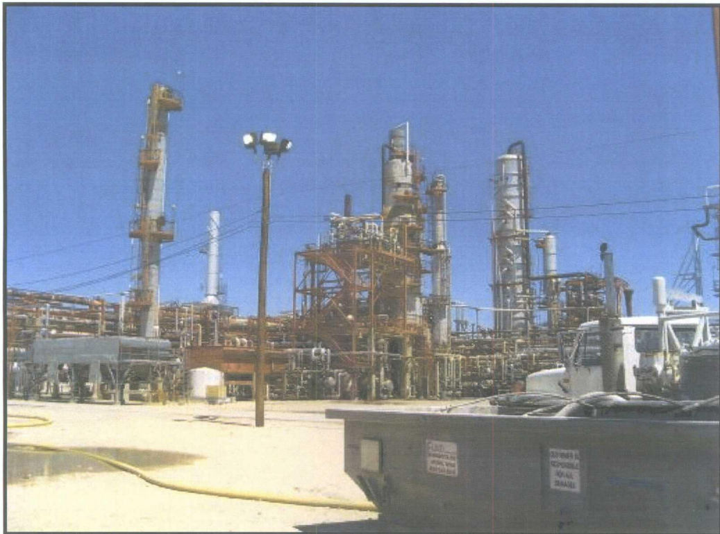
View from drilling area to process area, April 2009
