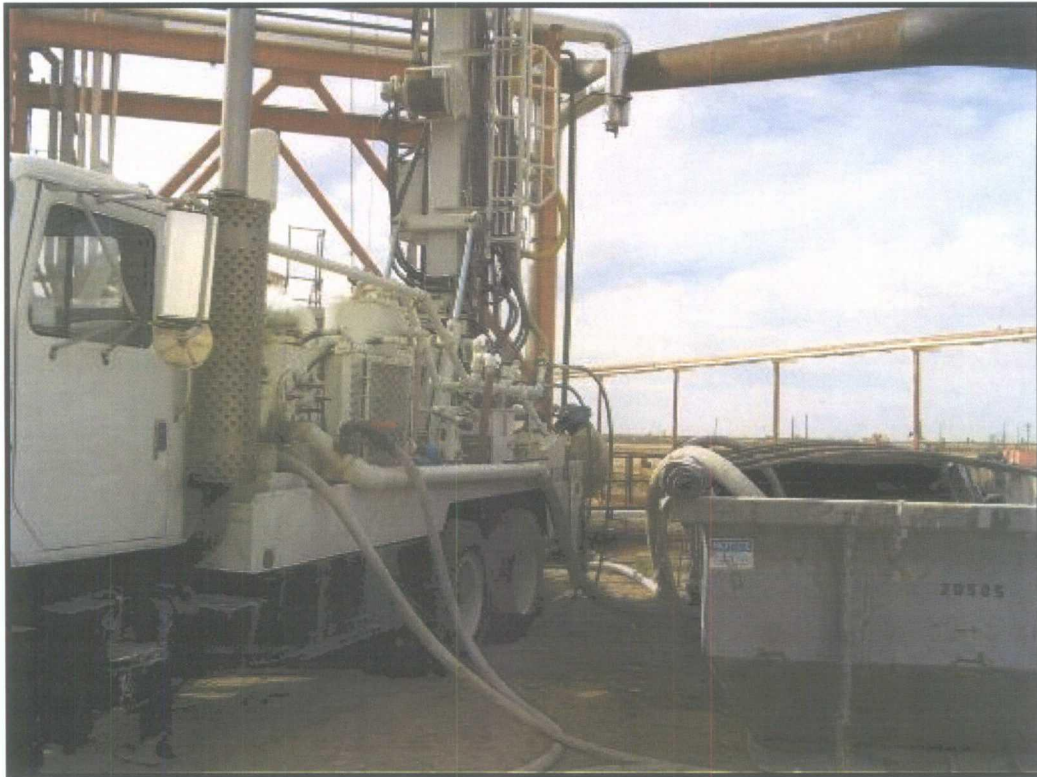
Drill rig and mud tank (plastic lined roll-off bin), April 2009
