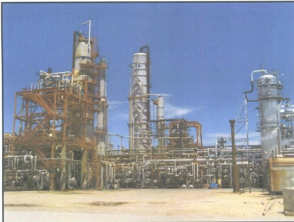
Looking northeast to refinery process area, April 2009.
