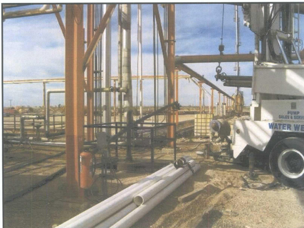
Drill rig positioned next to wastewater separator, April 2009
