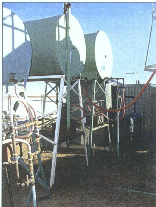
Photo 5: Install secondary containment underneath saddle tanks
