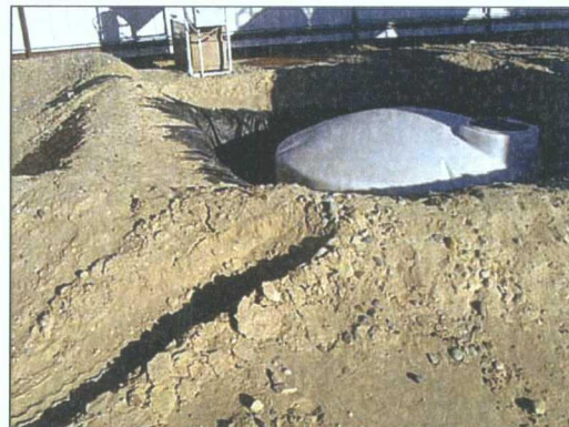
Photo 4: Repair Secondary Containment.
