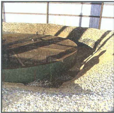
Photo 2: Clean out Sediment within secondary containment to expose side walls.
