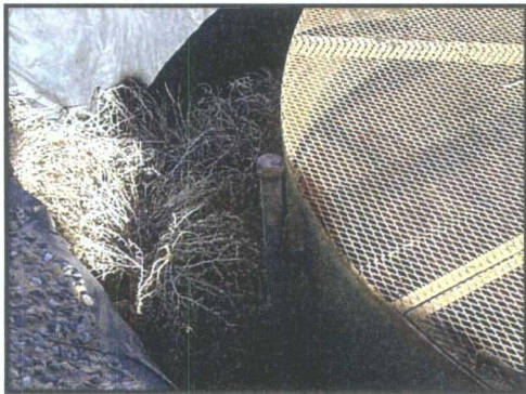
Photo 1: Clean out debris within secondary containment area.
