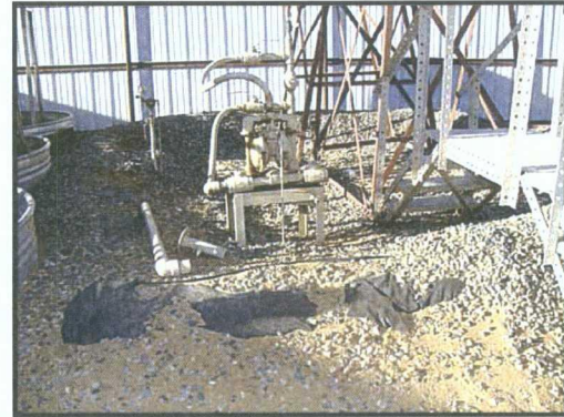
Photo 8: Repair Secondary containment.
