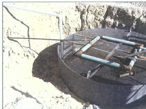
Photo 4: Below grade tank needs liners. Future plans to replace with an approved tank.
