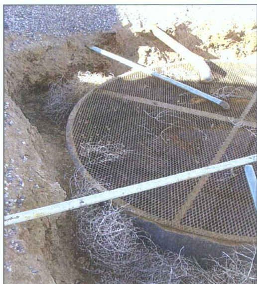
Photo 6: Clean out debris within secondary containment area to expose side walls.
