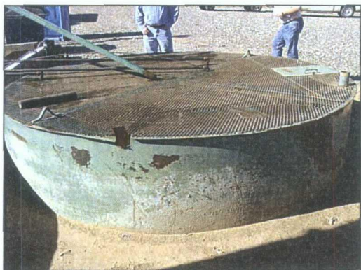
Photo 2: Install liner and properly sized secondary containment. For clarification this is not a below grade tank.
