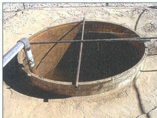
Photo 8: Below grade tank to be removed and replaced with an approved tank.
