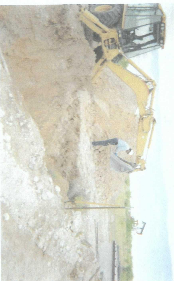
taking vertical sample with new, watertight box on right
